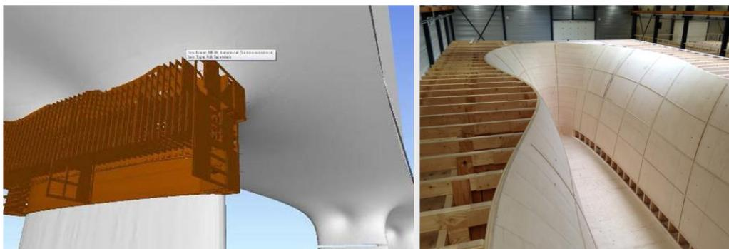
Figure 14: The timber formwork produced by Verhoeven Timmerfabriek for the supports of the bridge which is in the stage of realization by i-Lent
