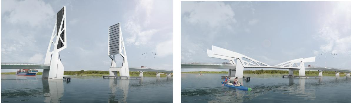
*Fig. 4.* The bascule bridge is a double leafed bridge
