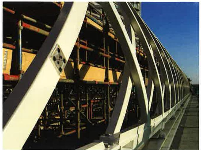
Fig. 8. Preparation for bolted connection prior to assembly (ZJA Zwarts & Jansma Architects)
